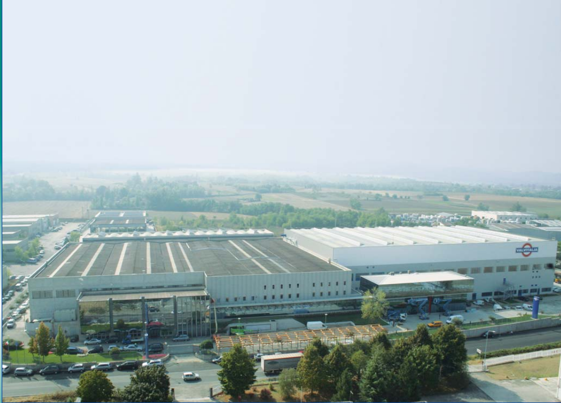
Rivanazzano (PV) Plant
